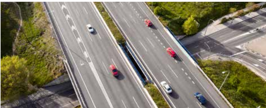
Technical issues: 'value engineering' by the private sector can sometimes result in construction defects, leading to penalties and deductions from the relevant government authority
